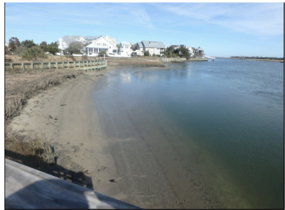
Fig. 15. Living shoreline location, facing north.
